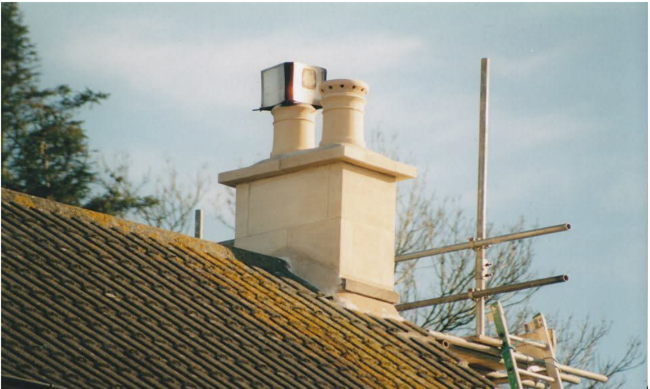
Two high-quality ashlar chimneys with differing styles of oversale (see p32)
